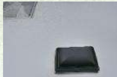
FIBERGLASS ROOF Durable, easy to clean (R-18) crowned fiberglass sheds water and doesn't cause black streaks like a rubber roof.
