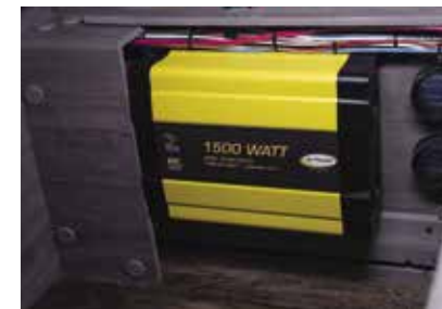
Optional 1500w inverter allows your battery-based system to run conventional appliances by inverting 12V DC to create 120V AC output. - N/A 2465
